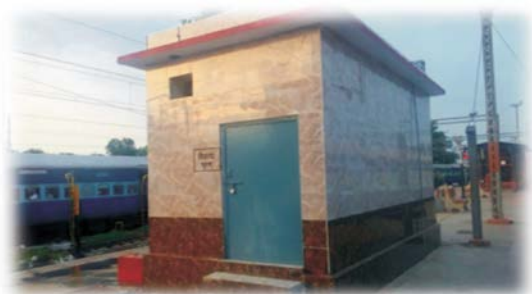
Toilet block at Varanasi railway station
